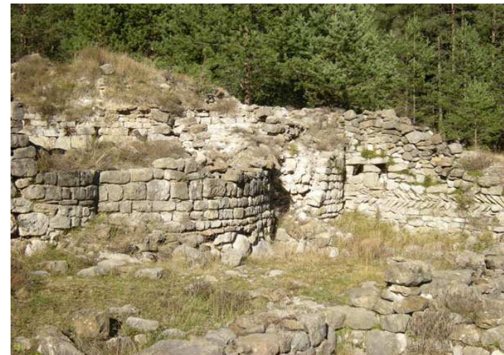
Hall annexed to the church. In the wall you see two inclined rows of flagstones in form of herringbone which is a type of construction used in the Romanic constructions.
